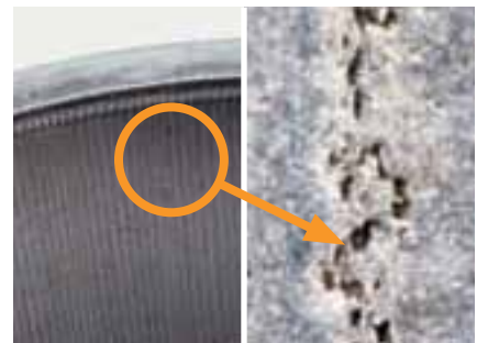
Fluting: Series of small axial burns caused by electric current passing through the bearing while it is rotating.
